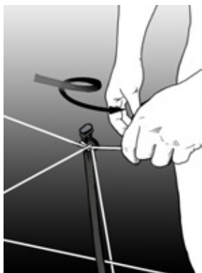
STEP 5 Tension wire and lock nut (clockwise). When creating a temporary paddock, place the reel post past the end post and complete by looping the top wire around the end post (5a). Finally, use guy ropes to straighten posts (5b).
