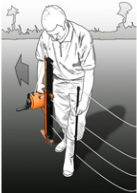
STEP 4 STEP 4a Place posts in ground as required. When a corner post is required, use a guy rope to ensure the post is straight (4a).
